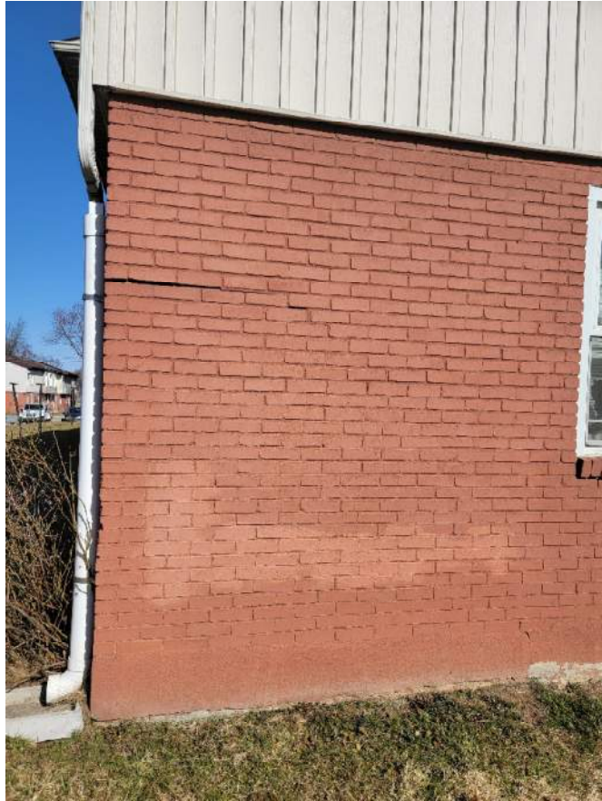
Typical historic rack and lateral displacement.
