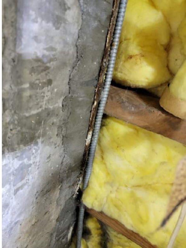
Cantilevered wood sill plate with mortar.
