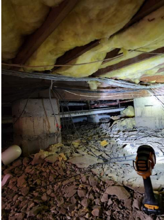
Typical floor joists bearing on center wood beam.
