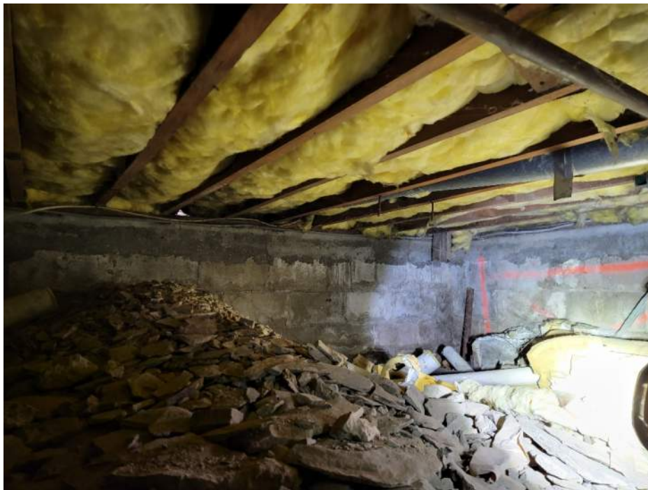
Typical floor joists bearing on exterior masonry wall.
