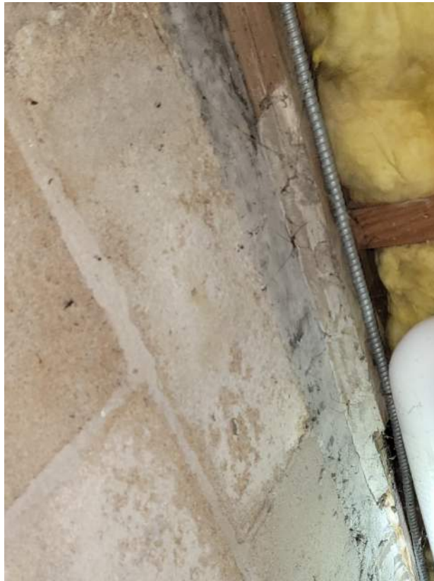
Cantilevered wood sill plate with mortar.
